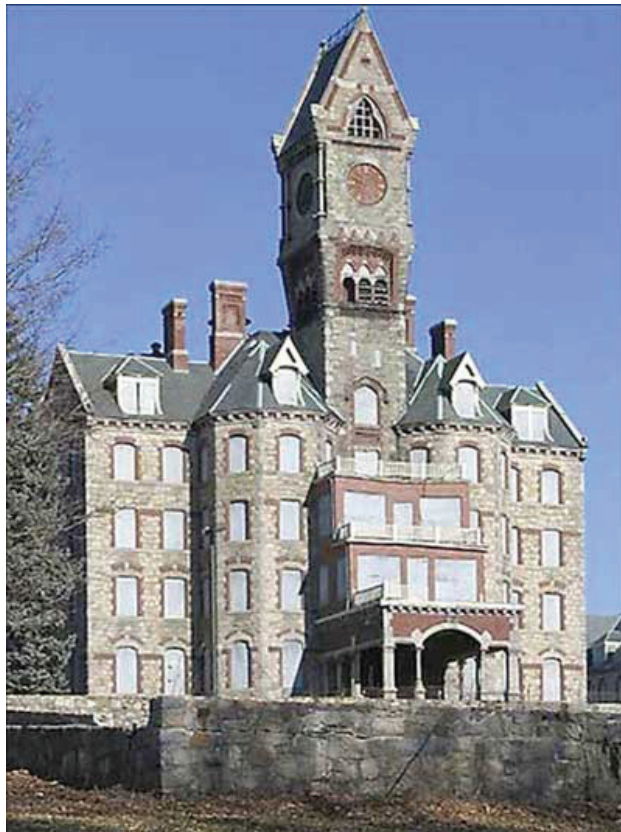
GOTHIC BUILDING — Preservation Worcester is working on a campaign to save this structure. Photo courtesy Preservation Worcester
