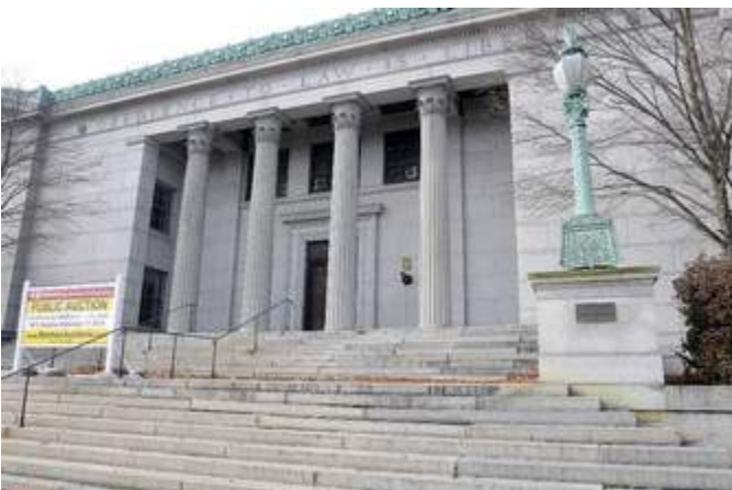
The exterior of the old courthouse.
