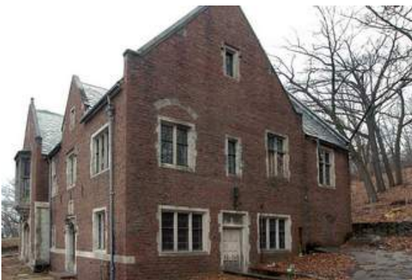
Fire Alarm and Telegraph Building at 224 Park Ave.
