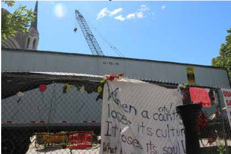
Crews worked on demolishing the Notre Dame church on June 25, 2018.
