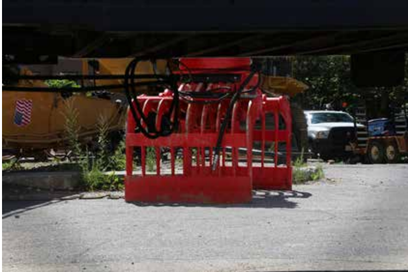
Demolition of the Notre Dame Church slowly continued on June 27, 2018.
