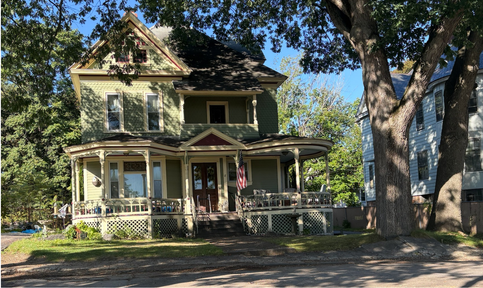
8 Melville St Site Visit-Built 1880
